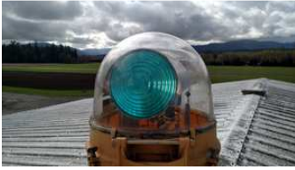
Crouse Hinds DCB-10 rotating beacon on top of the W28 maintenance hangar
