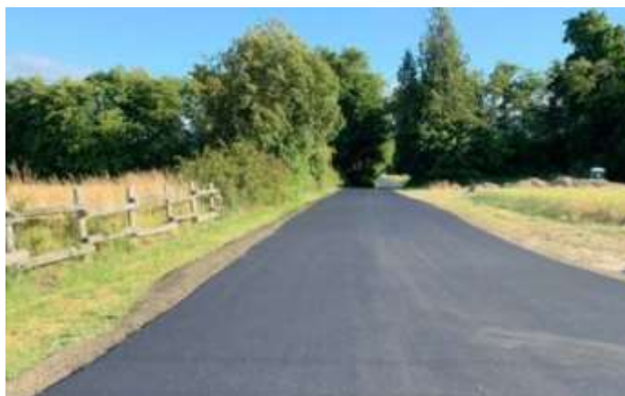
Newly asphalted entry road at Sequim Valley Airport
